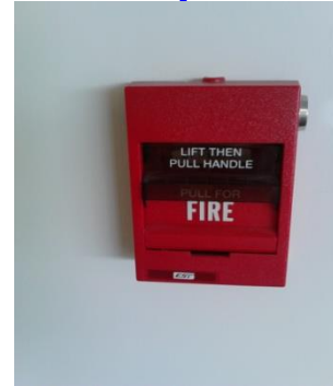
Fire alarm pull station
